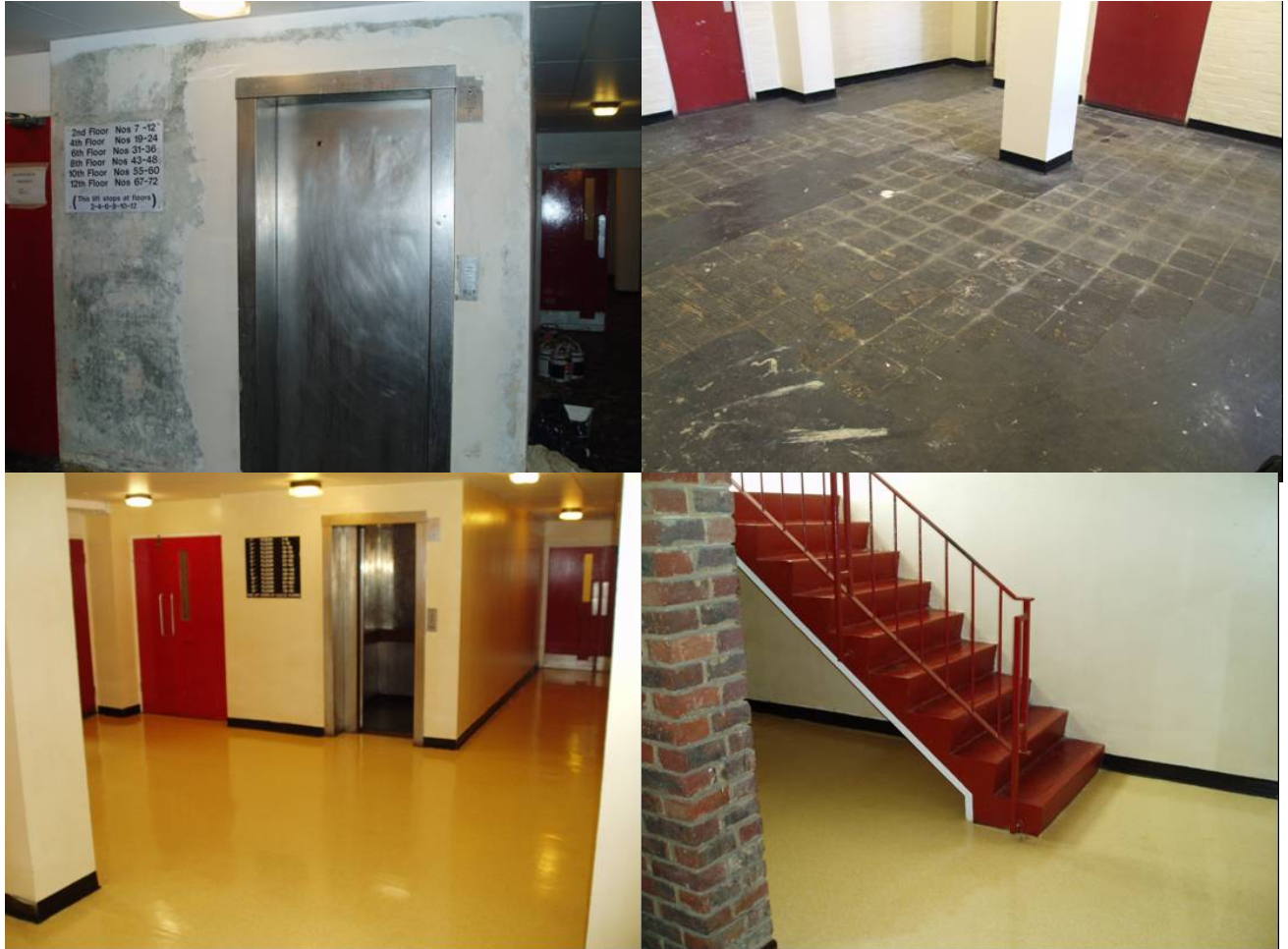
Transformed entrances to Franklin House, West Hendon - part of the Regeneration Estate Works programme for 2008/09.
